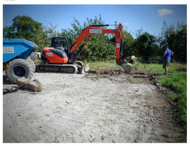
Plate 1. Removing grass and topsoil surfaces (looking SE)
